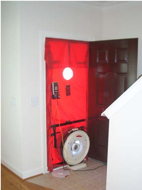
Figure 4 Blower Door set up unit 1204
